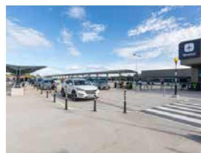
The drop-off and pick-up area with public transport bus bays in the background.
