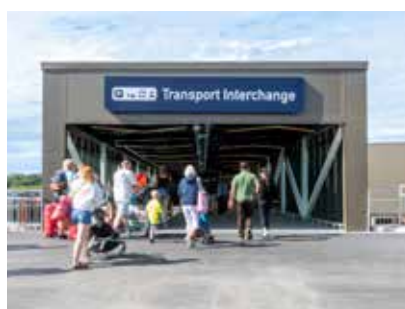
Link Bridge allowing customers to travel from the Terminal to the Transport Interchange.
